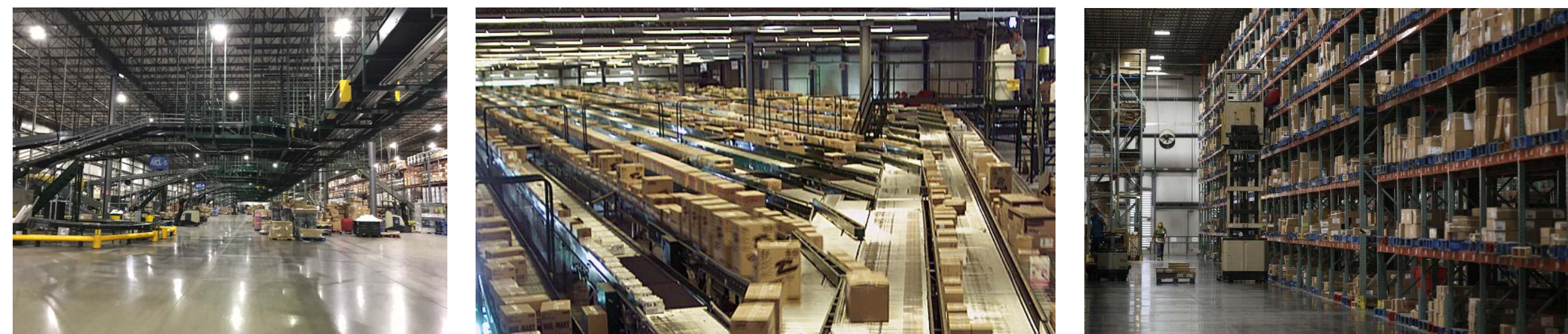
Figure 1. Inside a Walmart Regional Distribution Center.
